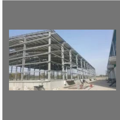
Box Type Industrial Shed
