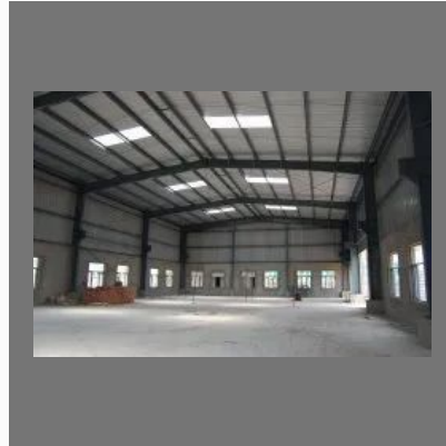
PEB Shed Construction
