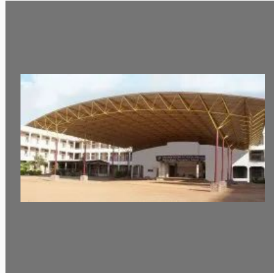
PEB Roofing Shed
