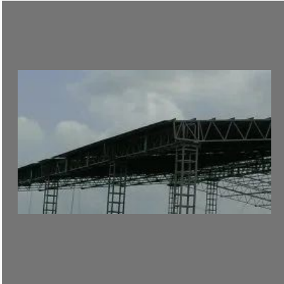
Industrial Shed Fabrication
