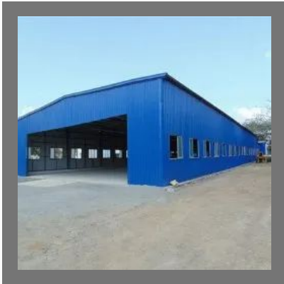
Mild Steel Roofing Shed
