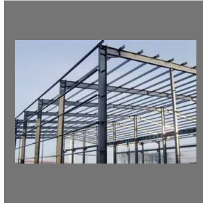
SS PEB Fabrication Shed
